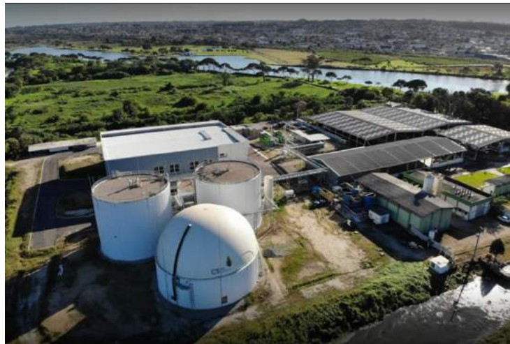
Figura 06 – Anaerobic digestion plant of CS Bio, Curitiba-PR.
